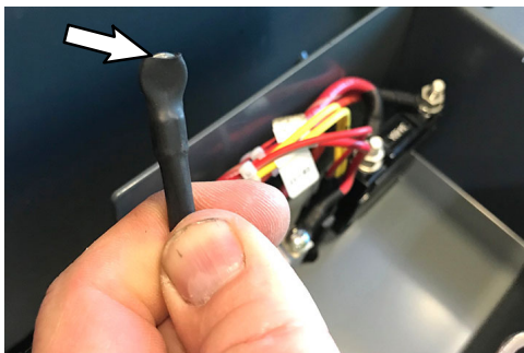
Fig. 3 - Terminal 150C NOT Properly Covered
